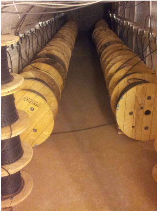
(a) Arrangement of cable drums
