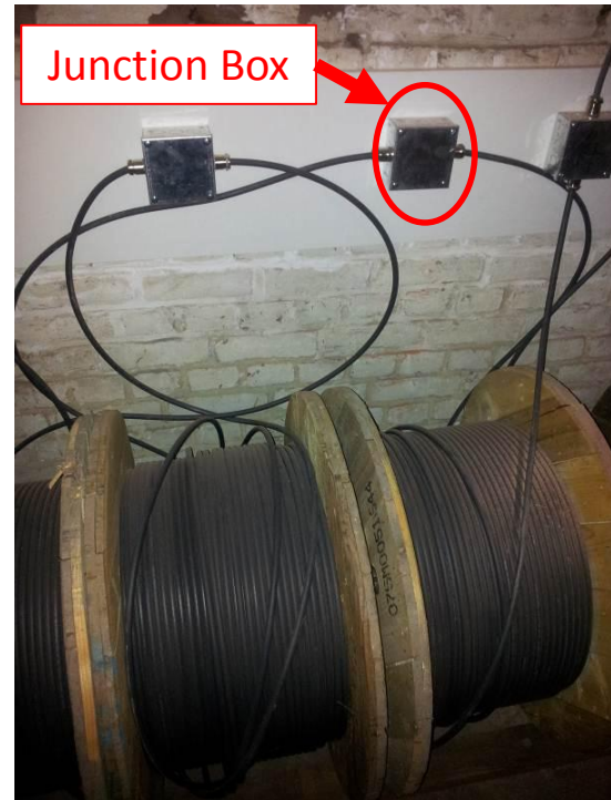
(b) Junction between two cable sections
